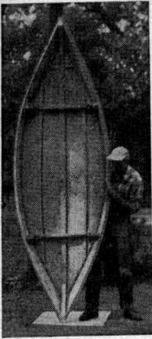
Fig. 4. Hull with bottom complete removed from form.
